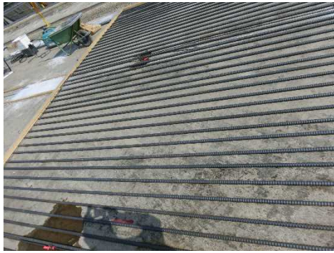
(a) 補強鉄筋 (D25@125)
